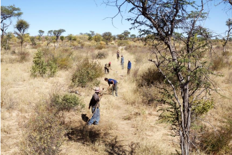
Building road to Den/ui.
